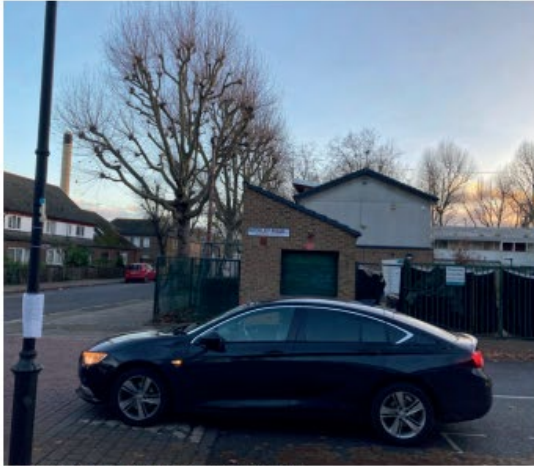
1 Looking south towards existing buildings on site
