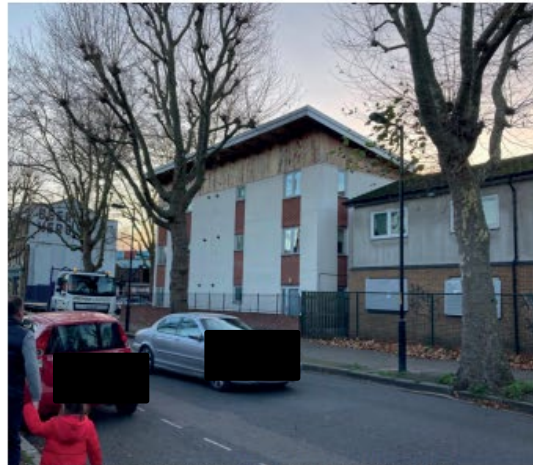
5 Looking southwest towards existing buildings on site and Georgia Court
